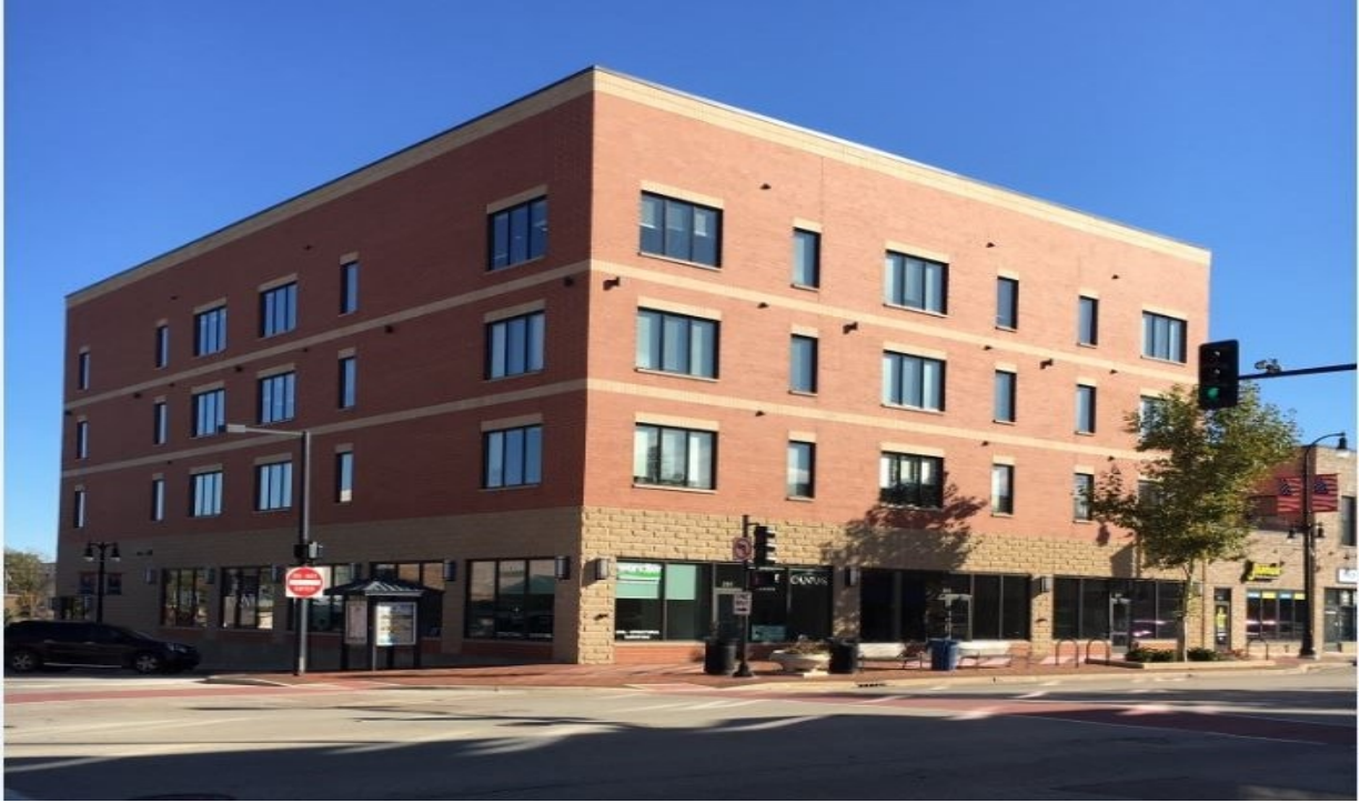
Plaza DeKalb—E. Lincoln Highway and Second Street
